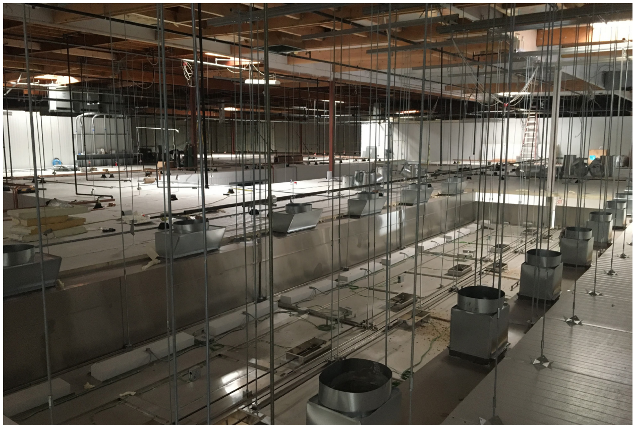
Construction of New Faber Street Foodworks Food Commissary
