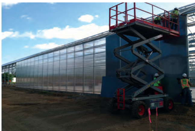
Green City Growers Cooperative, west wall panels under construction, August 2012. Photo: The Cleveland Foundation.
