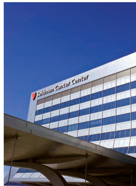
University Hospitals Seidman Cancer Center on the campus of UH Case Medical Center, constructed as part of Vision 2010. Photo: University Hospitals.
